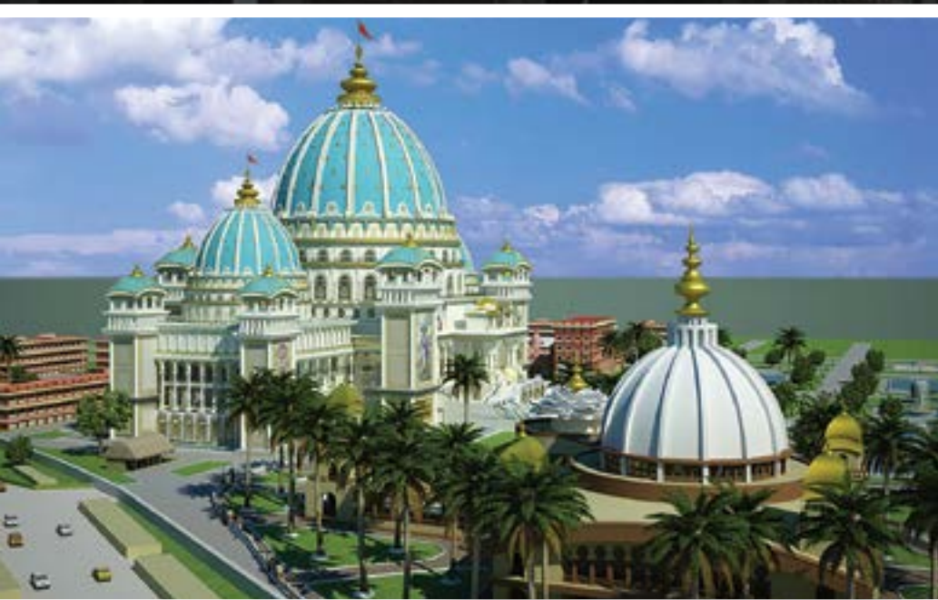
Workers atop one of the corner towers (main photo) help give a sense of the size of the structure, shown above in a computer-graphics illustration.
